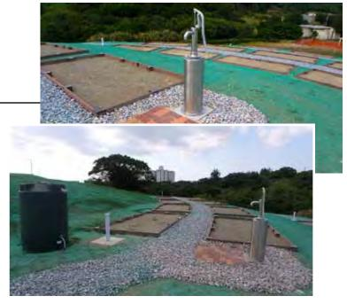
seen to the left. The Stainless Steel tank fills with water and is manually pumped out. The spout is equipped with a hose bibb for a water hose connection, or you can hang a bucket on the pail hook!
