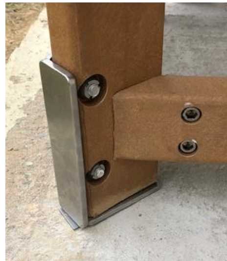
Photo 16 – Basin Table Anchor Nuts
