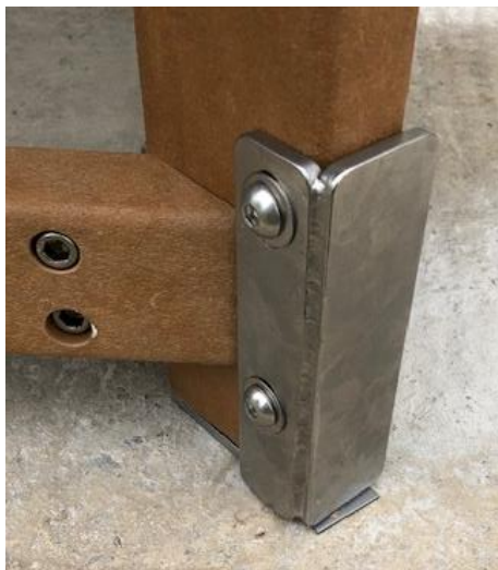
Photo 15 – Basin Table Anchor Bolts
