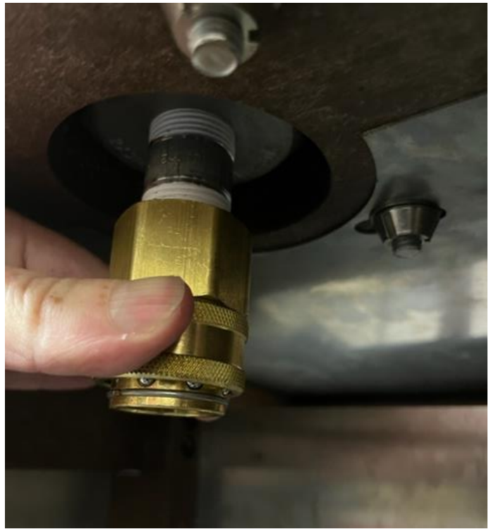
Photo 21 – Quick Connect Tank Connection
