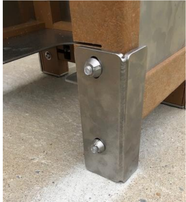
Photo 19 – Waterfall Table Anchor Nuts
