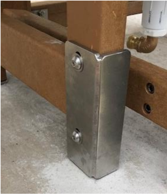
Photo 18 – Waterfall Table Anchor Bolts
